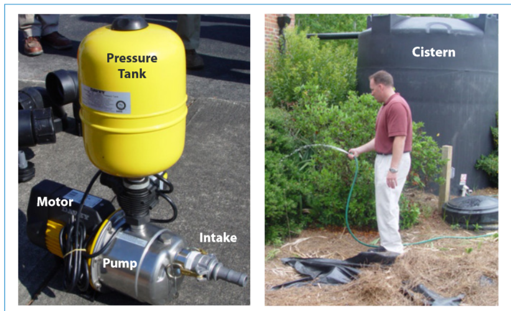
Figure 1. Pump with pressure tank before installation and example of system in use
